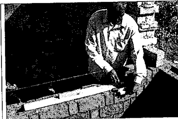
Image 2: Wooden tool while laying mortar
