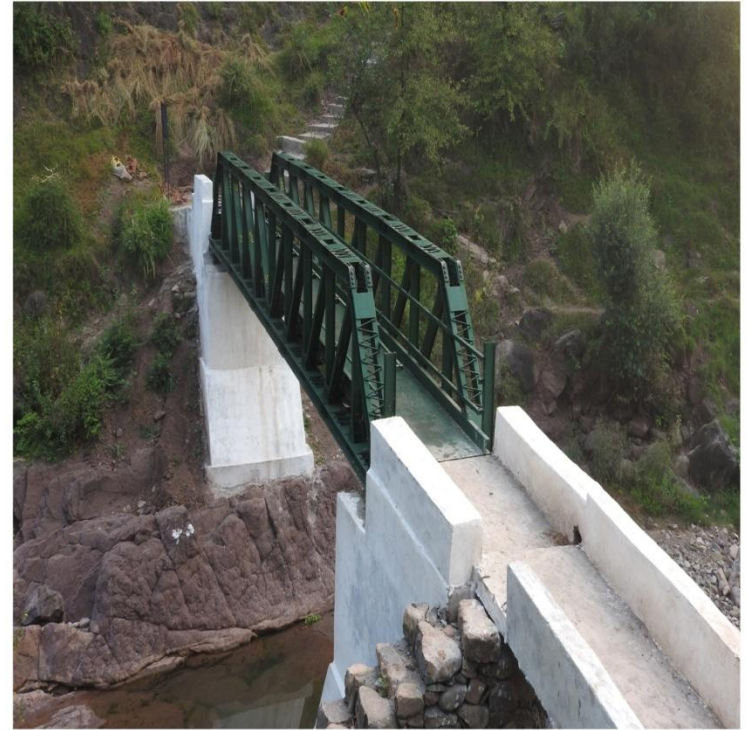
Constt. of Foot Bridge at Rajdhani Lower Panchayat: Rajdhani Lower E.Cost: 16.47 lac Scheme: MGNREGA Year: 2015-16 & 2016-17 Block: Manjakote Status: Completed
