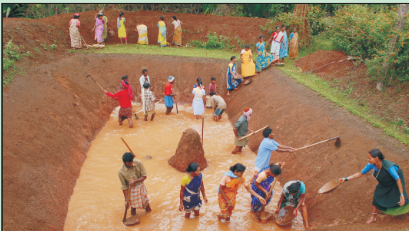
A Farm Pond Digging in Progress in Kottavalasa in Vizainagram District in Andhra Pradesh. The Day's Rain Water Is Deposited In The Farm Pond Created Under Mgnrega
