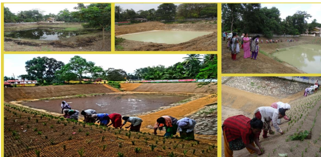
Image 1: Stages of Deepening and Desilting of Thiruvarmangalam Pond
