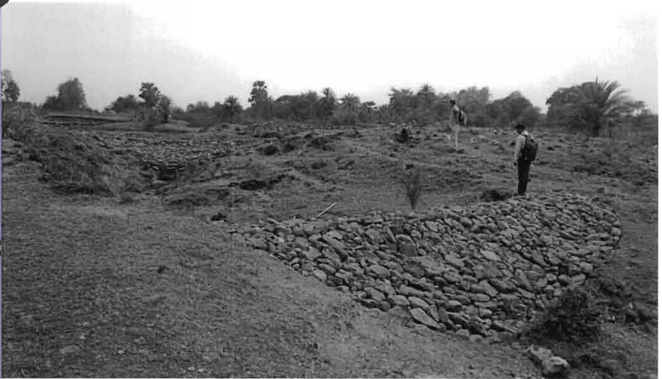
Loose boulder check in Littipara (Pakur)
